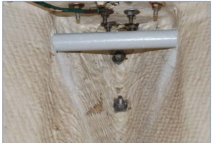
Fig. 2: Inside the hull showing the Hinge Tube installed
